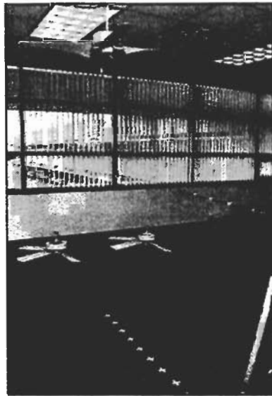
Figure 3. Air velocity test evaluates air moving efficiency at ½ ft. increments from fan center.
