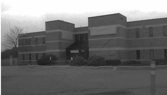
Figure 2 Elevation of the old infusion building. The infusion suite is in the wing on the right
