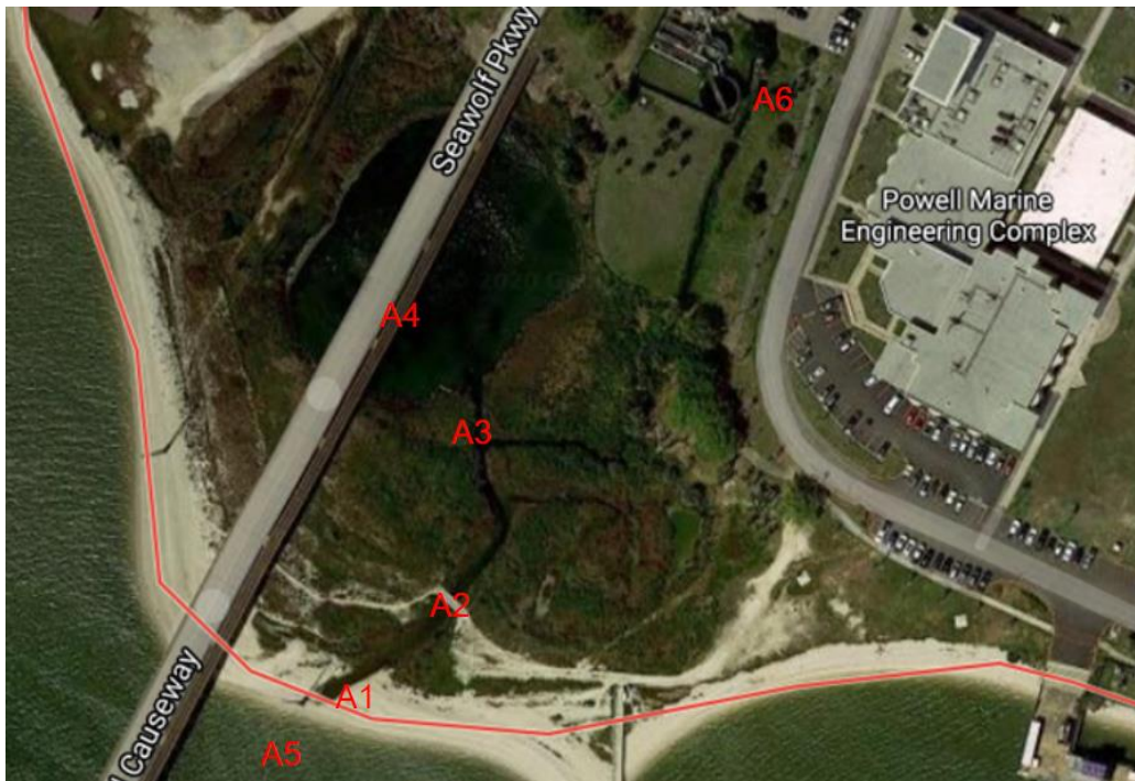
Figure 2: The wastewater treatment facility that is responsible for processing the wastewater of Texas A&M University at Galveston. There is a heavily vegetated marsh effluent stream that takes a longer route to the bay interface (A5). The shell beach face has a highly dynamic erosion/deposition cycle that can block the effluent stream from direct mixing of the stream and bay water.
