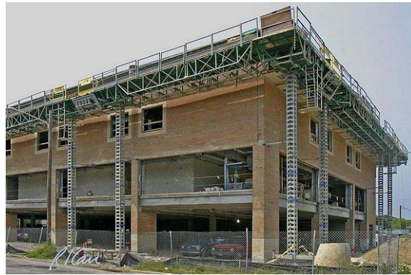
(b) Mast-climbing work platform
