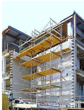
(a) Basic steel scaffolding
