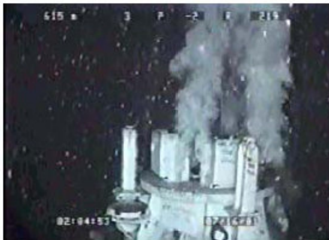
Fig. 2.5b- ROV photo of the TCRT on the Christmas tree surrounded by nitrogen gas bubbles from the SGN reactions. 10
