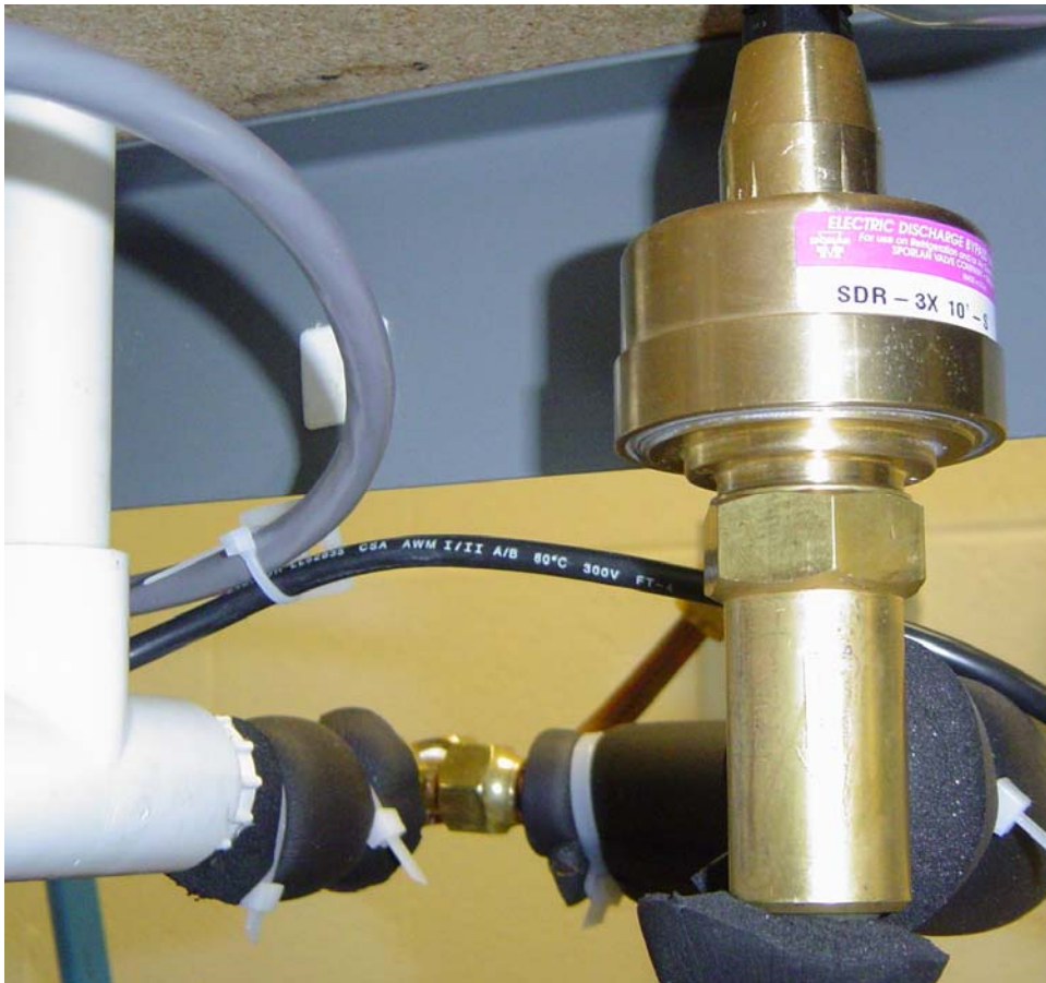
Fig. 2.15 Discharge valve (SDR)
