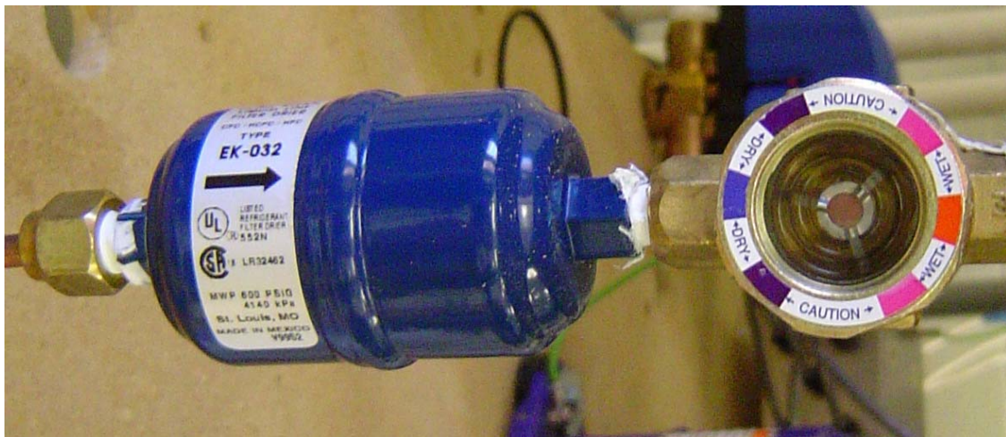
Fig. 2.20 Filter drier with sight glass
