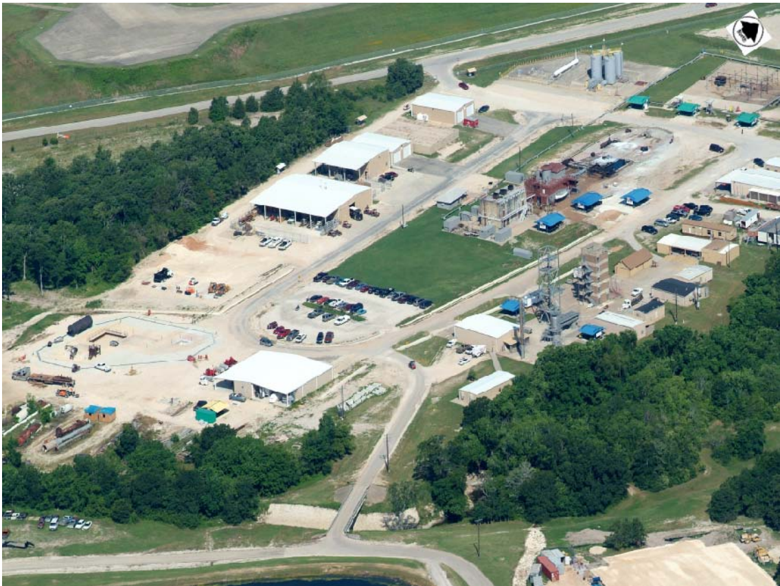
Figure 39. Aerial view of BFTF (courtesy of Kirk Richardson, TEEX)
