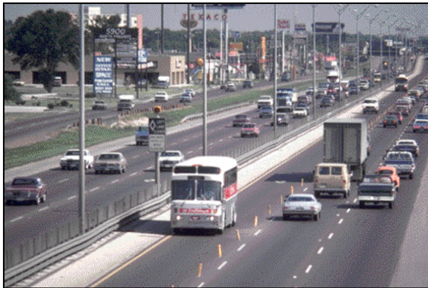
Figure 2.8. I-45 contraflow lane (Courtesy of TTI)
