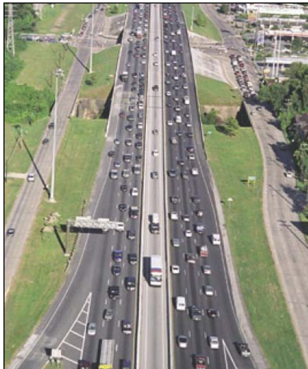
Figure 2.9. I-10 Katy Freeway HOV lane (Slotboom and Fuhs 2003)
