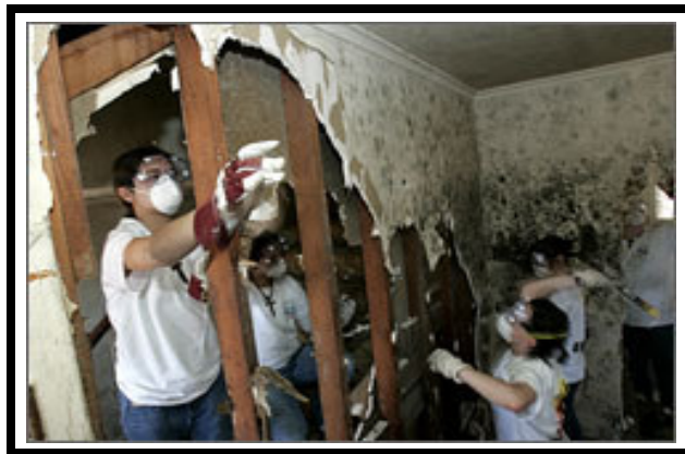
Figure 1. Mold remediation work following Hurricane Katrina (Szabo, 2006).
