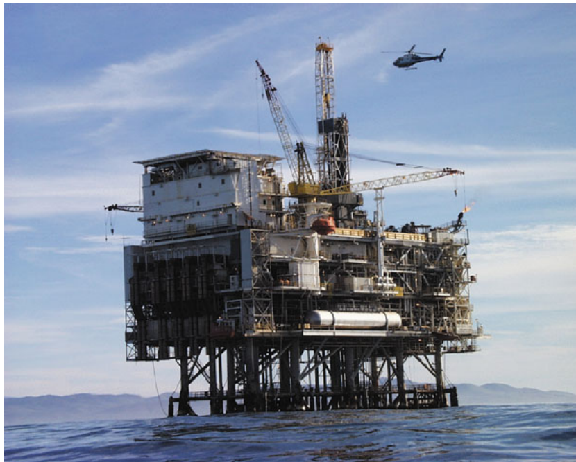
Figure 158. An offshore oil/gas platform ([102])
