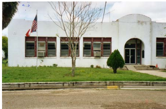
FIGURE 4. The La Vista High School After It Closed in 1994
