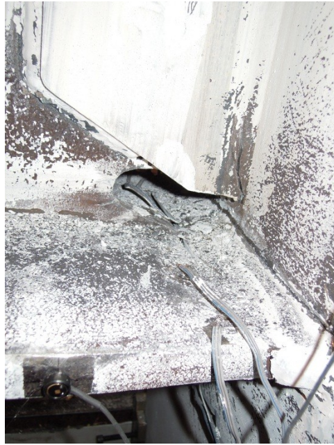
Figure 5.83 Photo of the east beam bottom flange of Specimen 4 after the first loading cycle of 7% drift ratio
