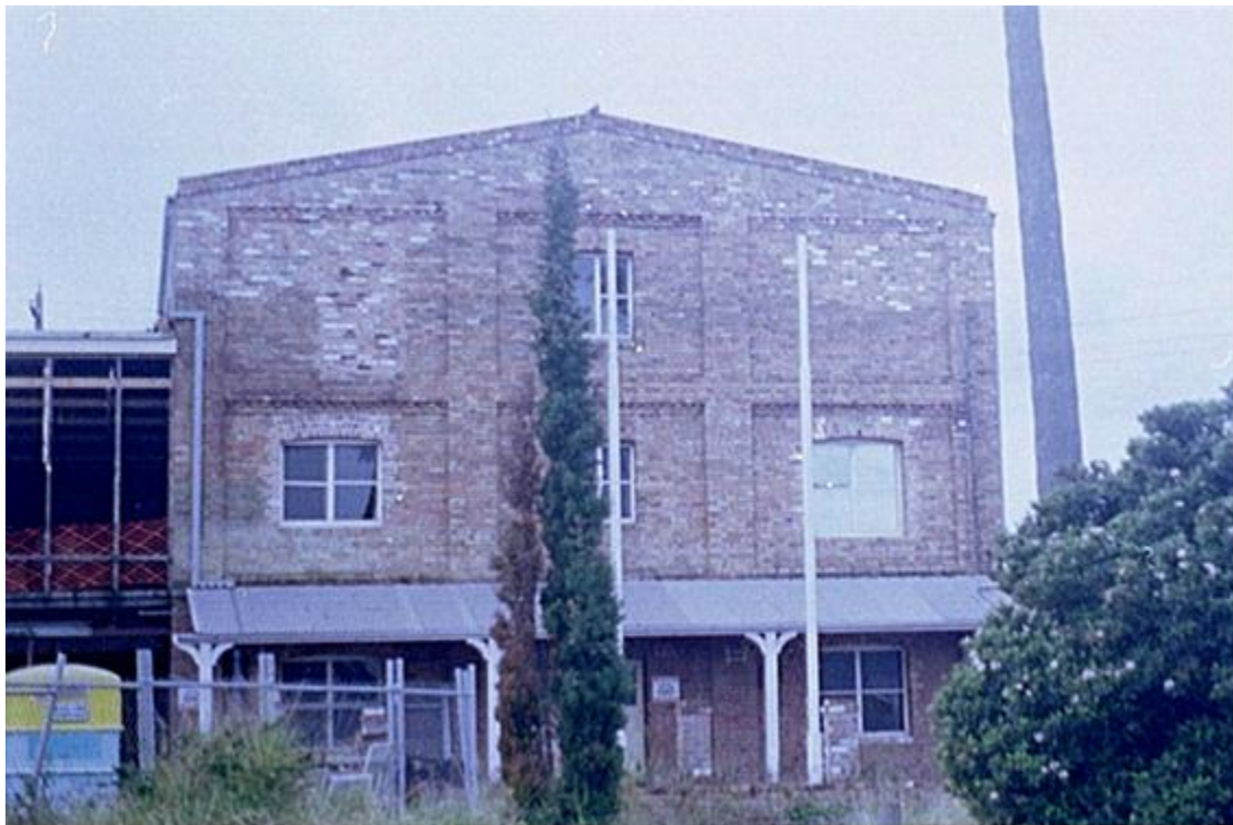
Figure 3 Flour Mill damaged in 1989 Earthquake, courtesy Nichols (1999)
