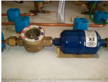
Figure 2.9: Filter/drier
