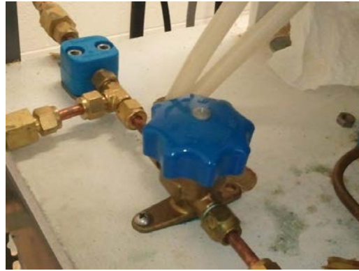
Figure 2.7: Manual shutoff valve
