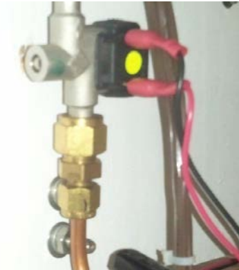
Figure 2.6: Expansion valve
