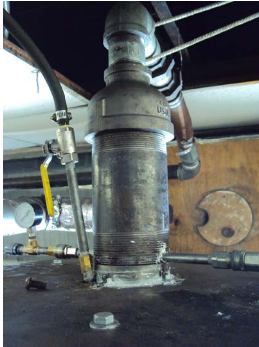
Figure 23: Boiler plate assembly
