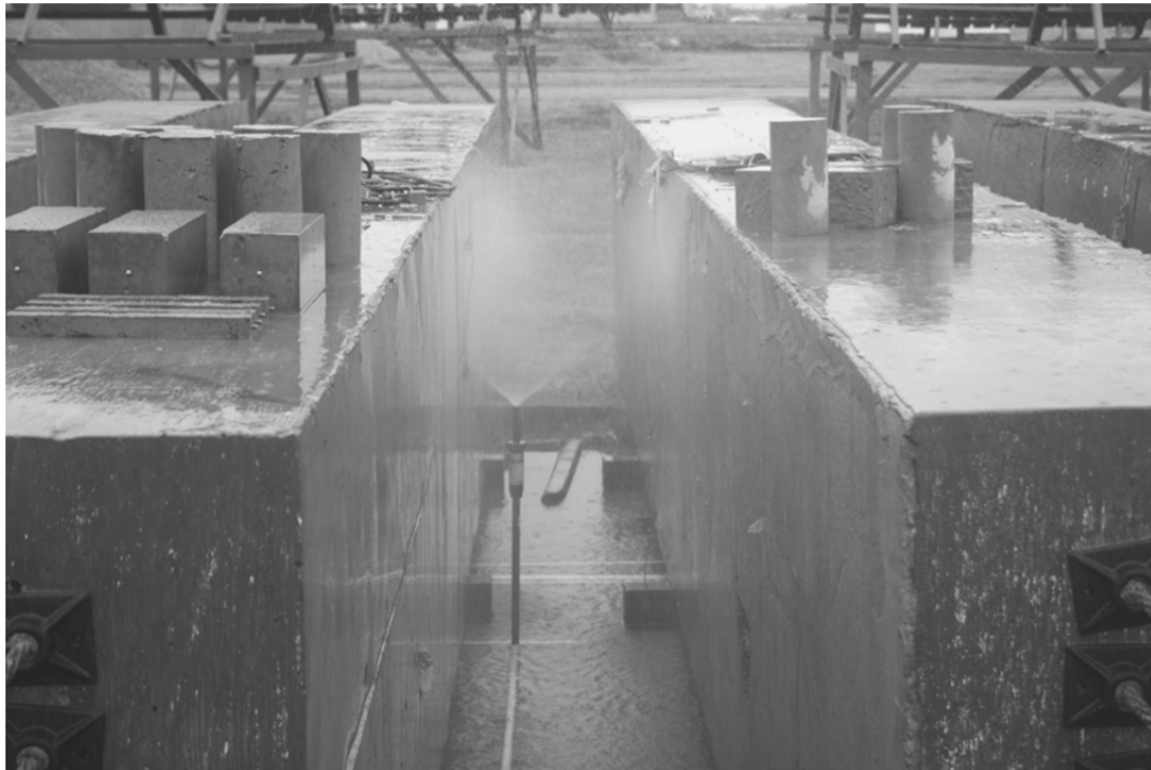
Figure 3-4. Sprinkler System between Two LSC Specimens [taken from Alberson (2009)].
