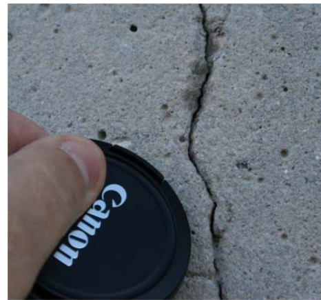
(b) Close-up View of a Typical Crack
