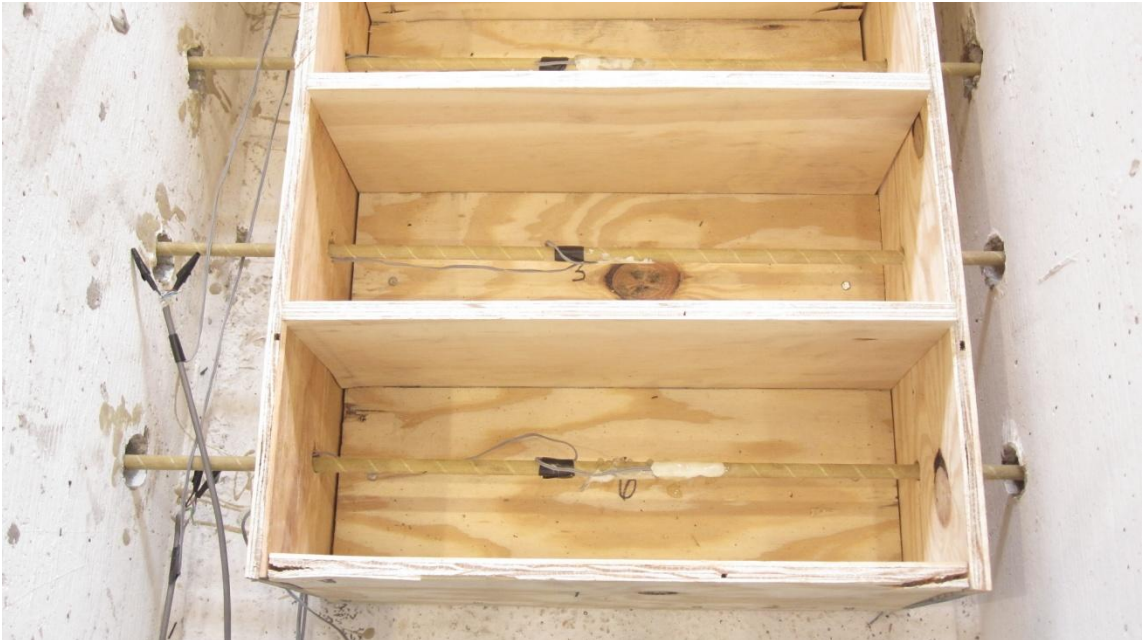
Figure 74 Formwork for concrete to encase bars
