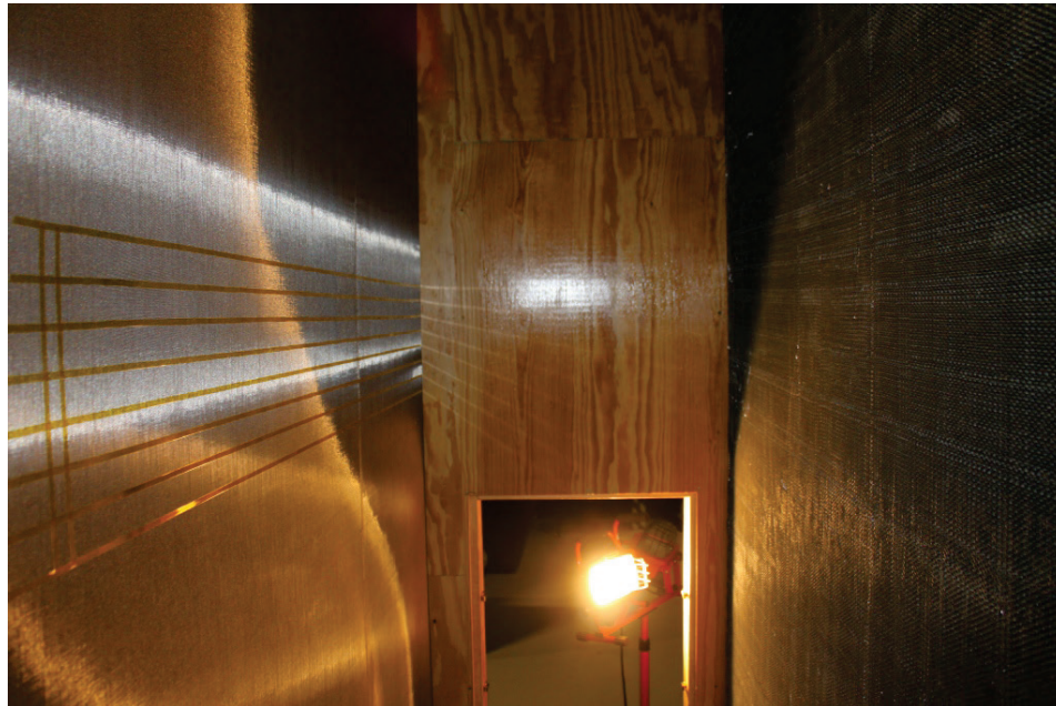
Figure 8-3. Tape on upstream side of screen one (flow moves right to left from this angle).
