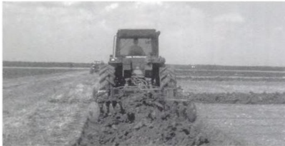
Figure 8. Rice levee construction with a levee plow. Source: Smith, C.W. and R.H. Dilday
