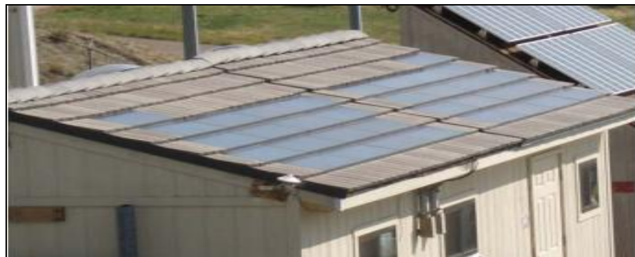
Fig. 1 The 2 kinds of mounted PV roofs. (Source: Muller et al. , 2009)
