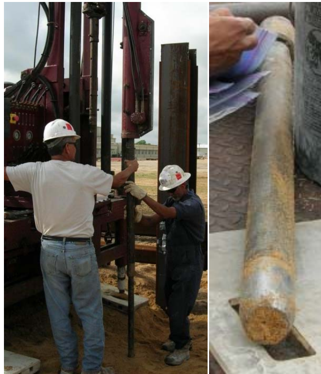
Figure 3.9. Standard penetration test (SPT) on loose sand and split spoon sampler
