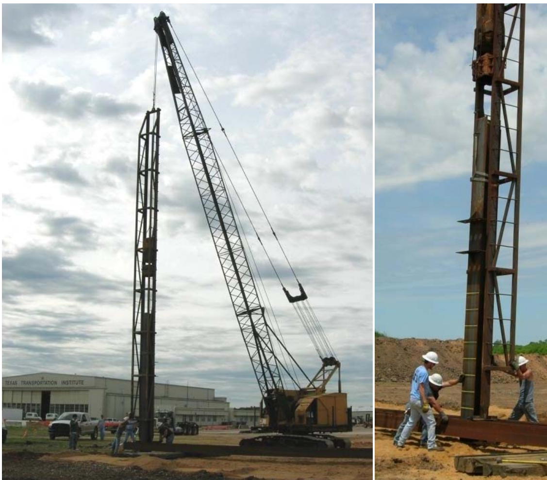
Figure 3.152. Pile driving rig and pile driving into the loose sand ditch
