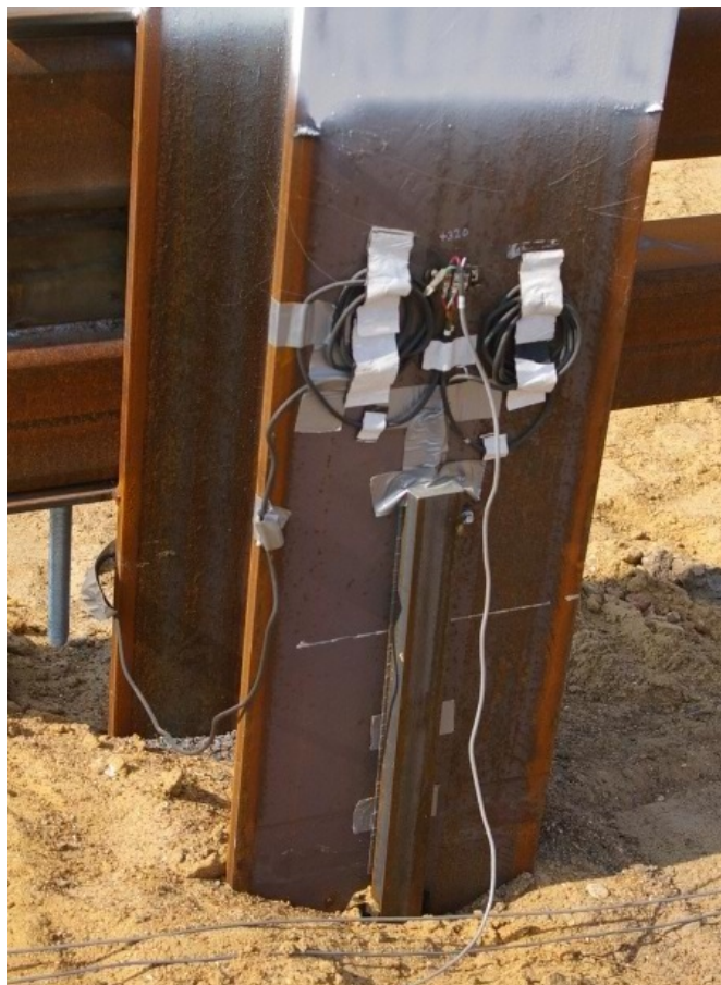
Figure 3.158. Strain gage attached on the post
