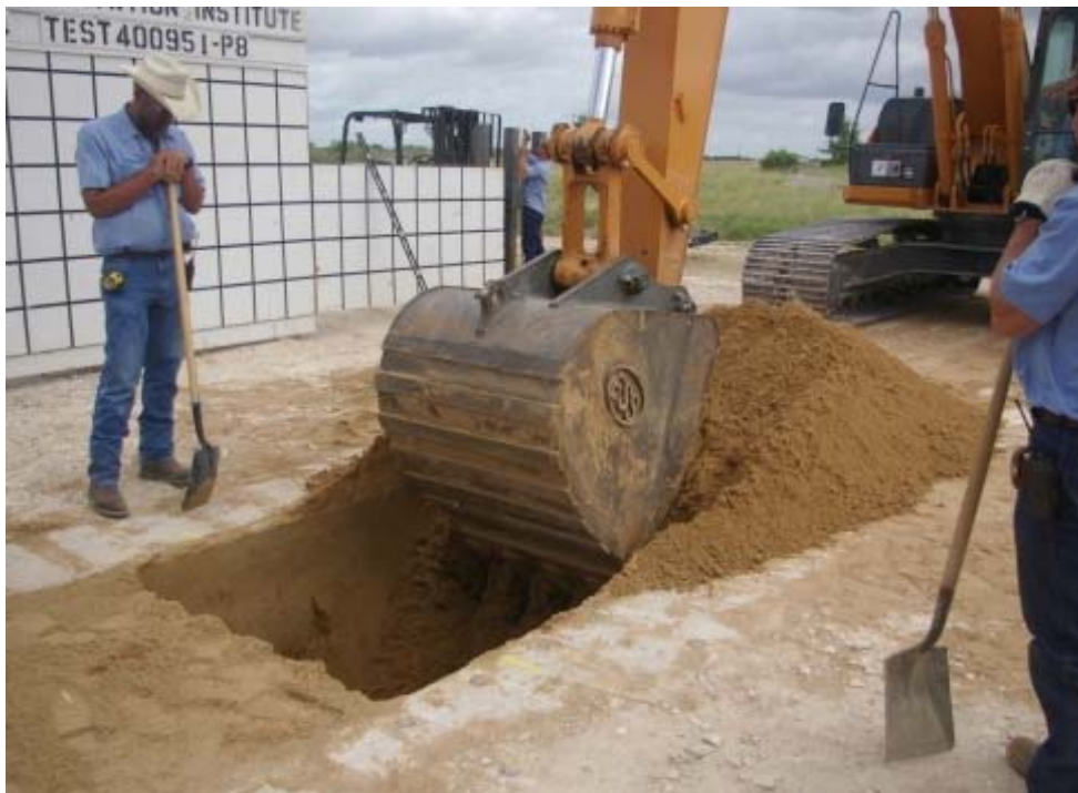
Figure 3.72. Excavation of the loose sand pit to install the posts system
