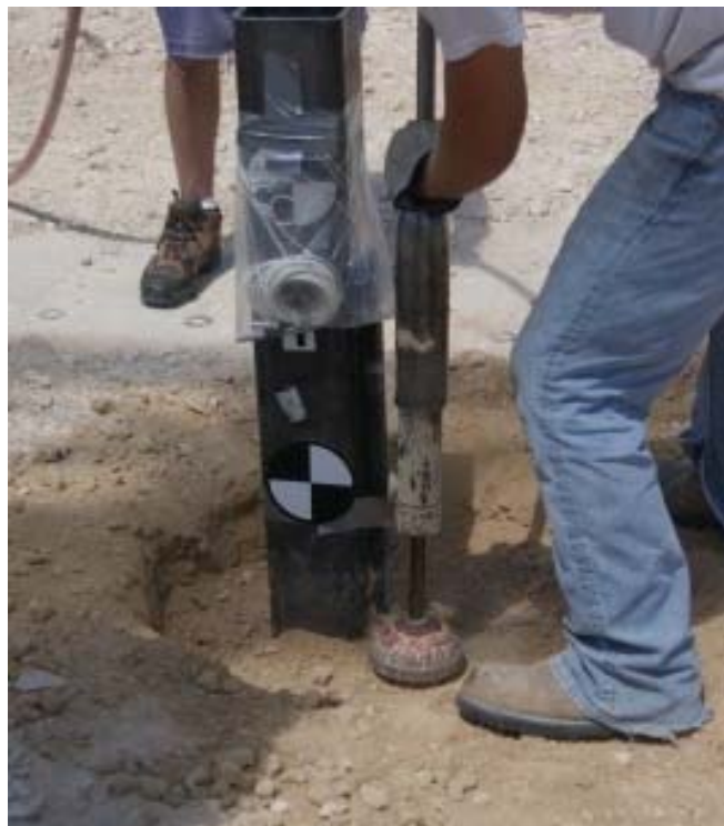
Figure 3.48. Soil compaction during the post installation using a mechanical tamper
