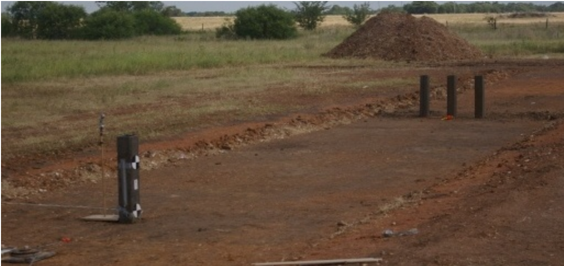
Figure 3.125. Single post and group of posts system embedded in hard clay
