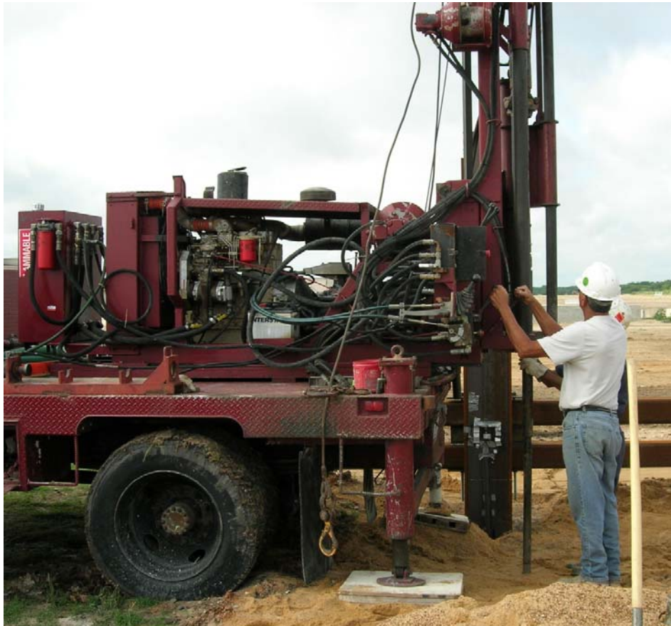
Figure A. 1 Standard Penetration Test (SPT)
