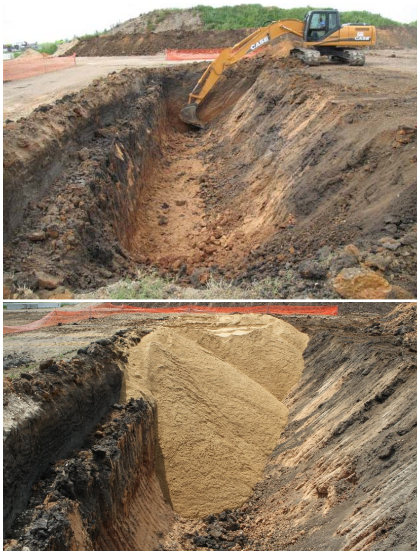
Figure 3.151. Loose sand ditch construction
