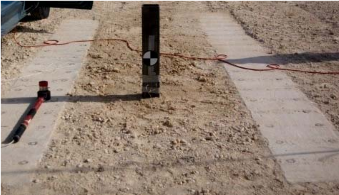
Figure 3.49. Post after the installation
