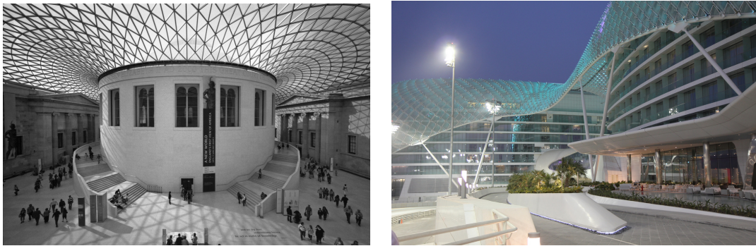
Fig. 3. An example of triangulated (left) and quadrilateral (right) glass panels (©Drew Leavy (left) and Sakena (right)).
