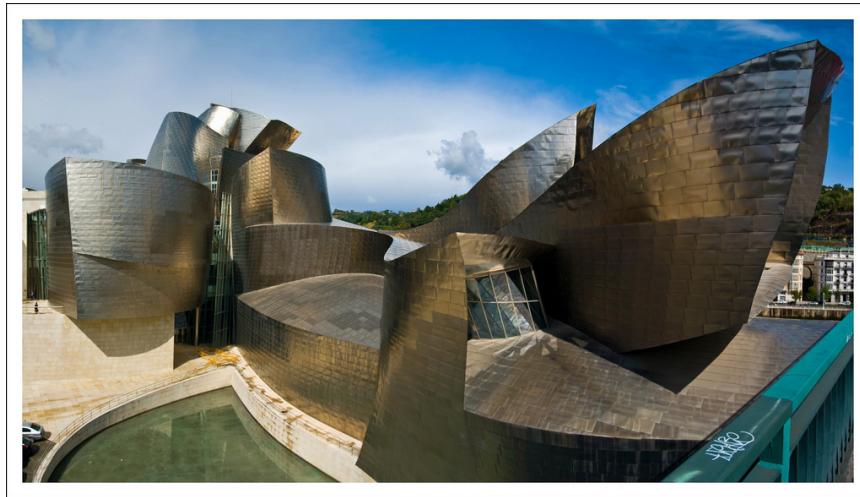
Fig. 2. Guggenheim Museum Bilbao, Spain is an example of free-form architectural design using developable surface (©Bastian).
