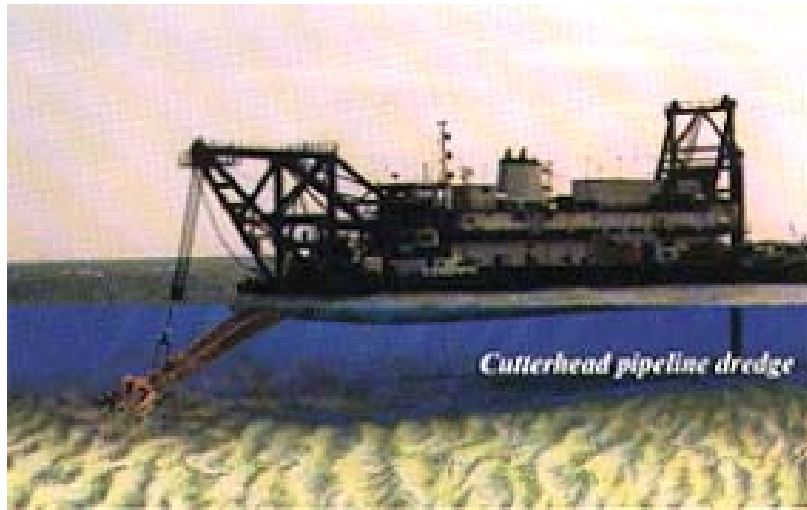
Fig. 1. Cutterhead pipeline dredging channel bottom( U.S. Army Corps of Engineers ).
