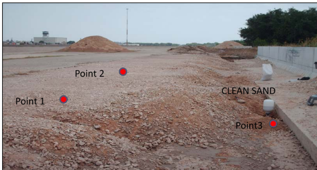
Figure 8. Field Area Tested on MSE -Wall (Riverside Campus, Texas A&M University)
