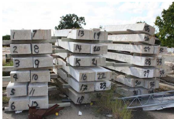
Fig. 26. Storage positions of GFRP reinforced beams
