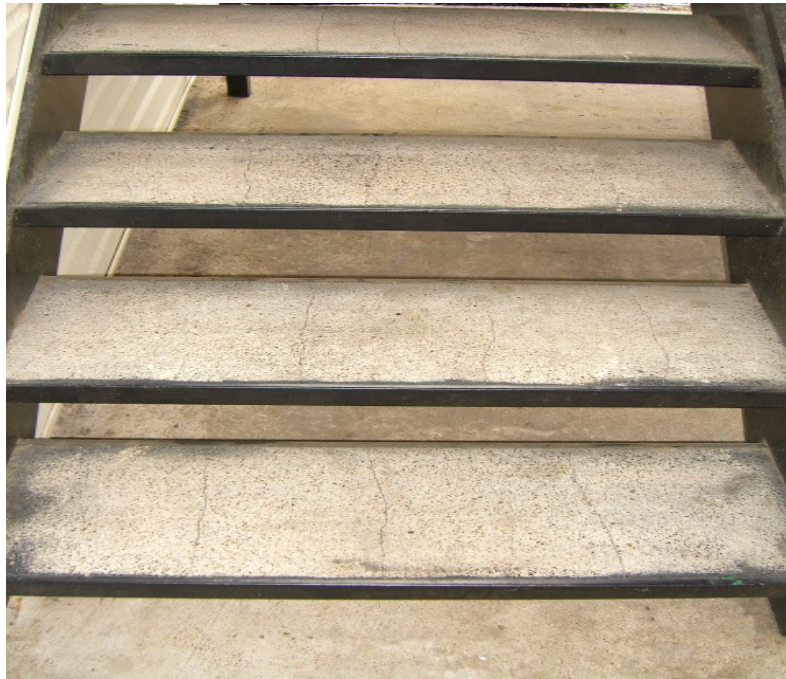
Figure 53. It is hollow between two stairs. Because MV used micro-switch to do the mechanical interaction between MV and stairs, this type of stairs can not be climbed by MV. The reason is that micro-switches can not touch the wall of stairs since they are mounted in front of MV. The micro-switches help MV to decide when ball screw should come out.
