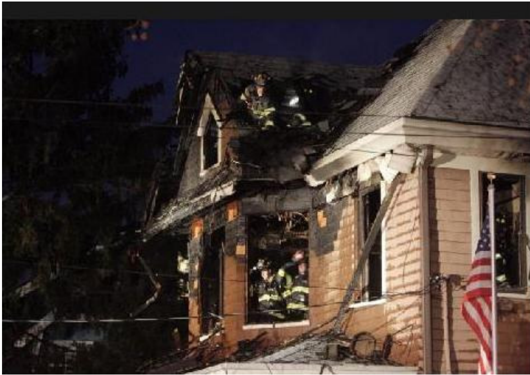
Figure 1. Firefighters check the inside and roof after the fire is extinguished. ( http://www.silive.com/news ) (Advance Photo/Bill Lyons)
