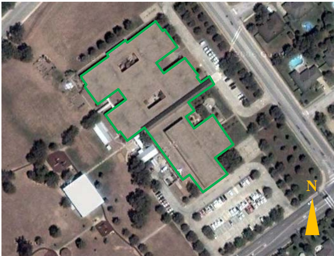
Figure 4.2 - Satellite View of the Case-study School (Source: http://maps.google.com )
