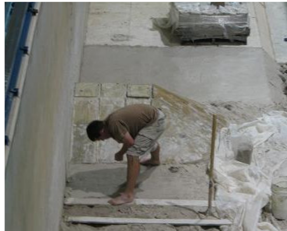
(b) Plaster work
