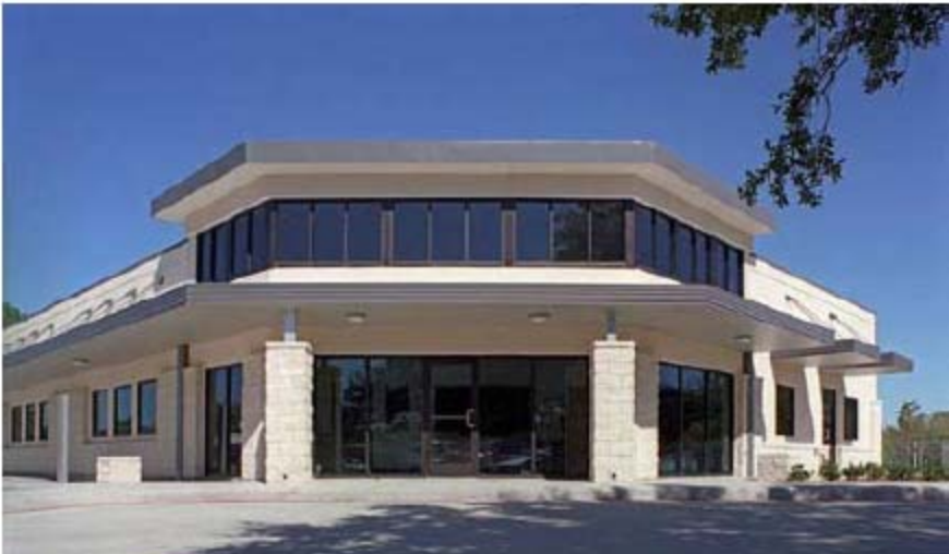
Figure 91: Pearlman Pediatrics Exterior Image of windows and external shading devices Source: Haggard J. Photography
