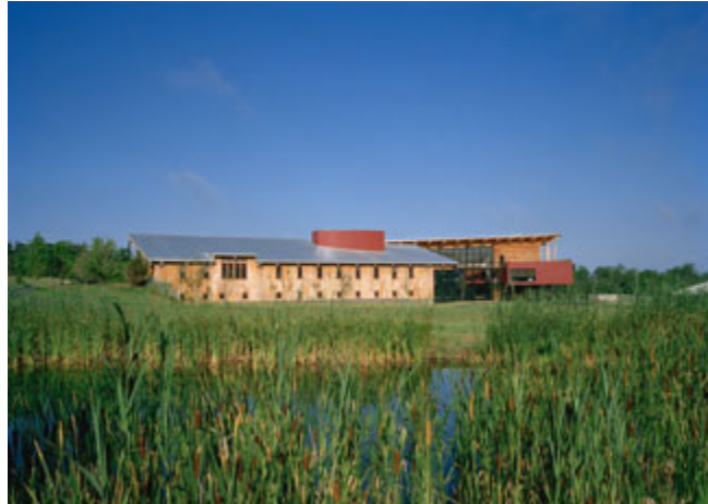
Figure 5: The Patrick Dollard Discovery Health Center Case Study Image of Facility and Surrounding Landscape Source: Guenther, R.
