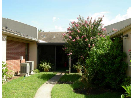
Figure A-13 The courtyard providing insufficient space to walk
