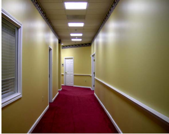
Figure 4-1 Example of handrail that is not easy to hold on
