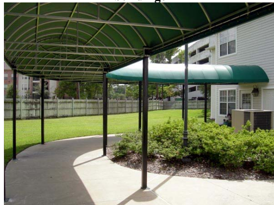
Figure A-23 Covered walkway connecting two main buildings
