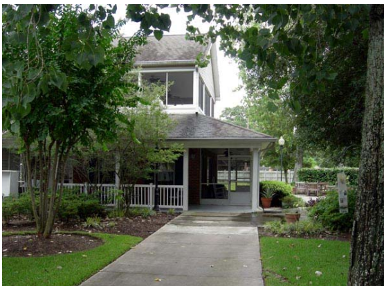
Figure A-22 Outdoor walking path of PG assisted living facility
