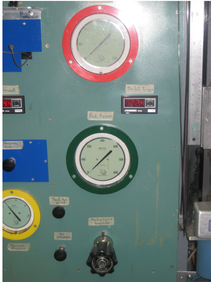
Fig. 3.5—Part of panel showing inlet and outlet pressure gauges and back-pressure regulator at bottom.
