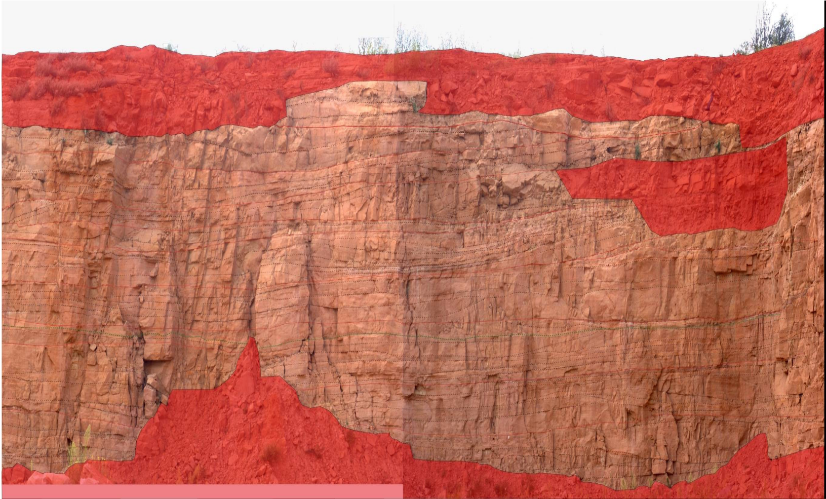
Figure 1-8: CarmeuseNA quarry South wall part 8. Far western side of South wall.
