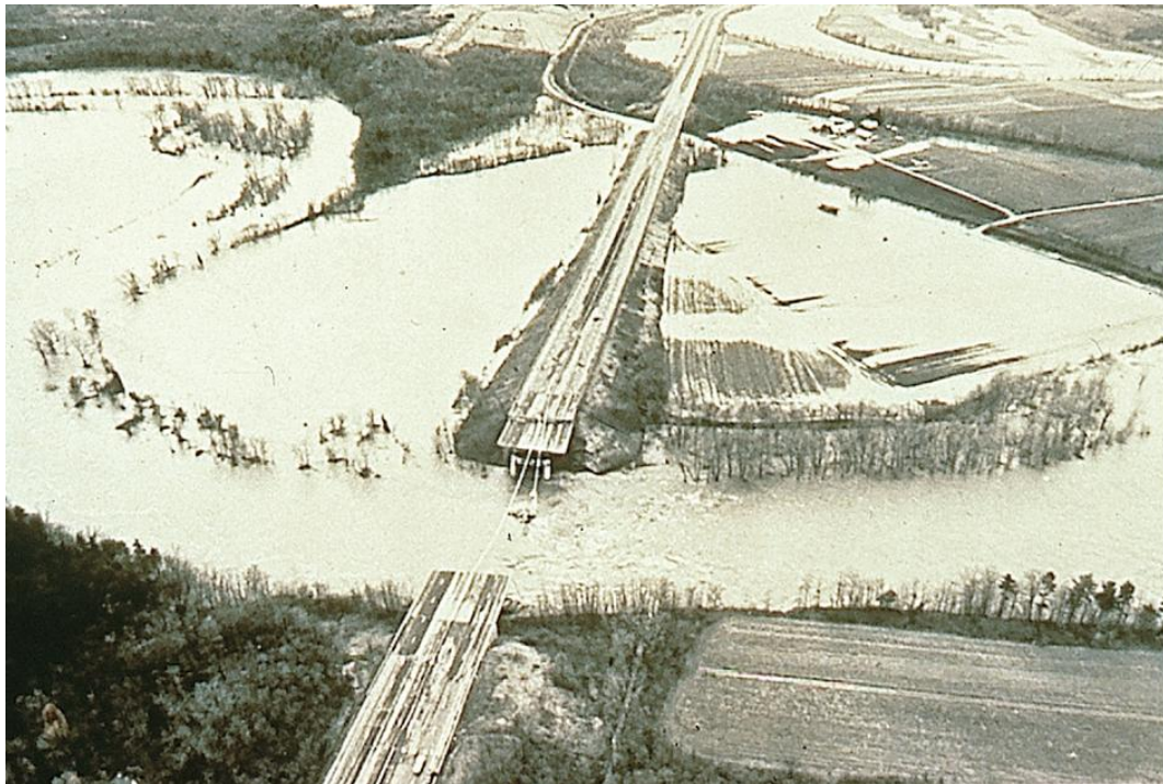
Figure 7-4. The 1987 Schoharie Creek Bridge failure.
