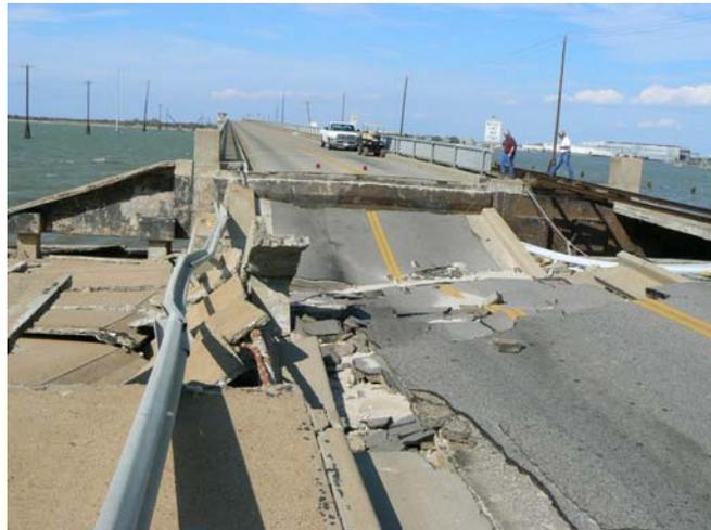
Figure 1.3: Damaged Pelican Island Bridge at Galveston, Texas by Hurricane Ike in Sep. 2008
