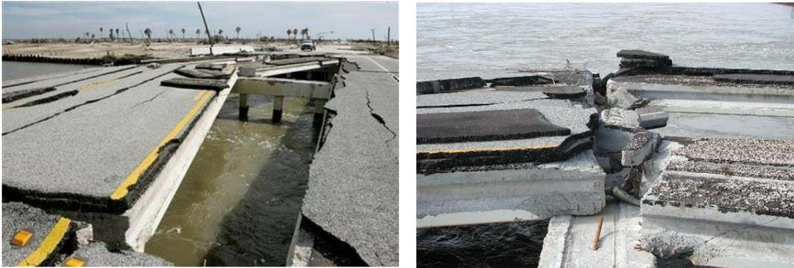
Figure 1.4: Damaged Bridge at Rollover Pass, Texas by Hurricane Ike in Sep. 2008
