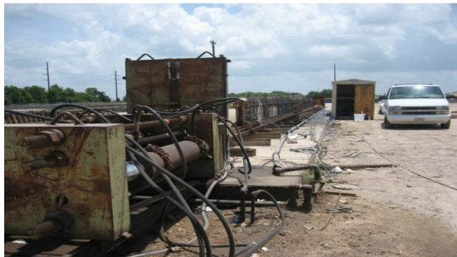
Figure 4.17. Prestressing Bed with Strands.
