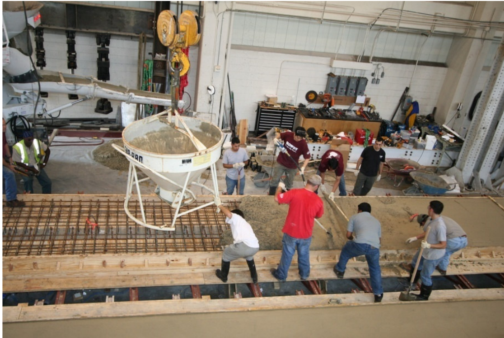
Figure 4.20. Placement of Deck Concrete.
