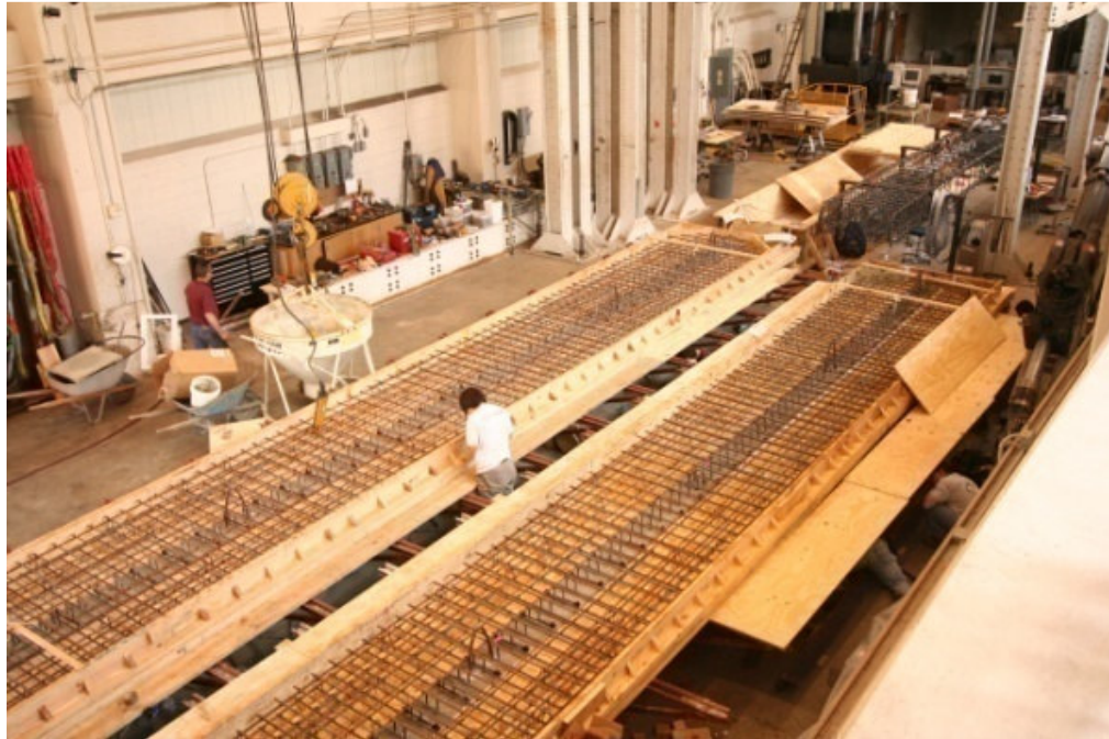
Figure 4.19. Placement of Reinforcement.
