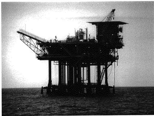
Figure 5. High Island 389 platform. The superstructure is located 1.5 km east of the coral cap of the East Flower Garden Bank in the northwestern Gulf of Mexico. The above-water structure functions as a steel island, providing roosting sites for migratory birds transiting the Gulf of Mexico.
