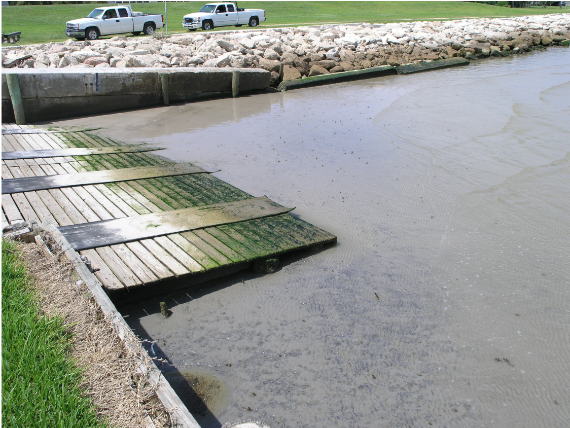
Figure 50. Sediment building up at the Camp Casa Mare marina. Picture taken on 14 August 2006.
