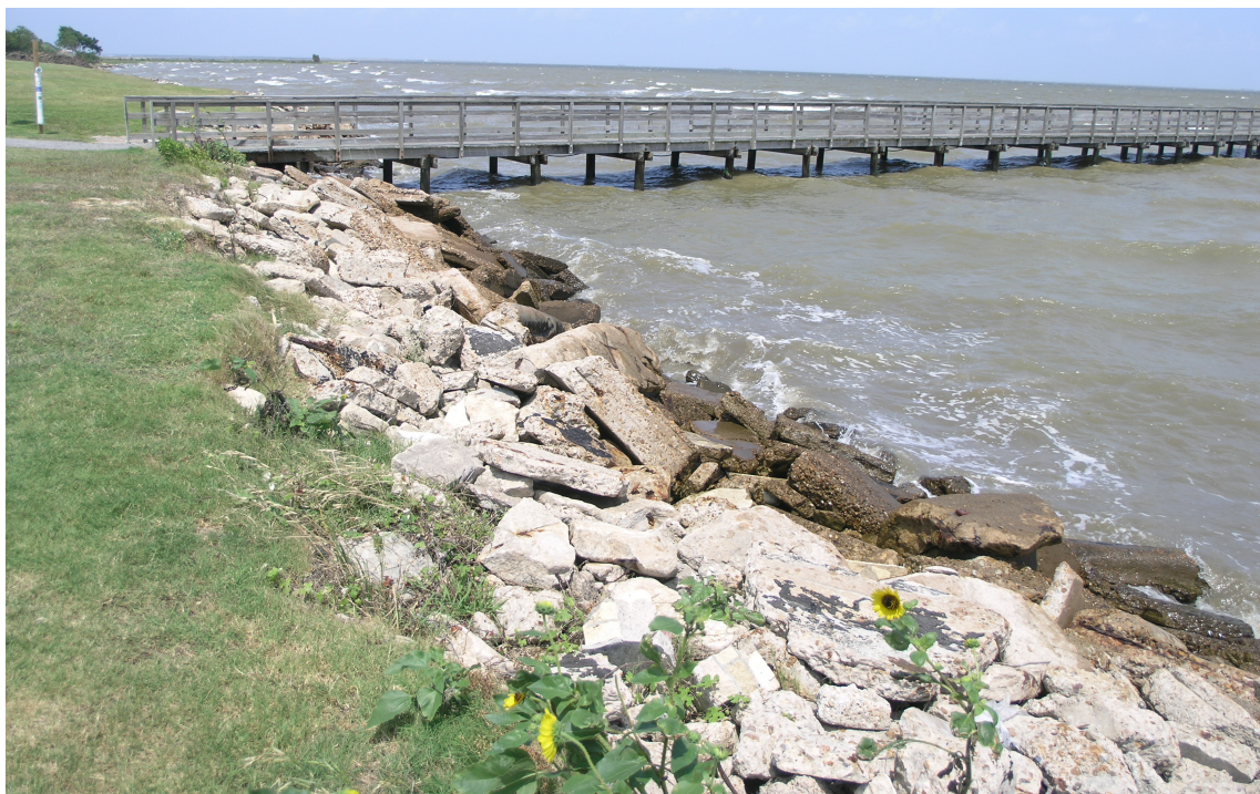
Figure 10. Shoreline armoring with concrete rip rap. Picture taken at Pine Gully Pier, March 2005.
