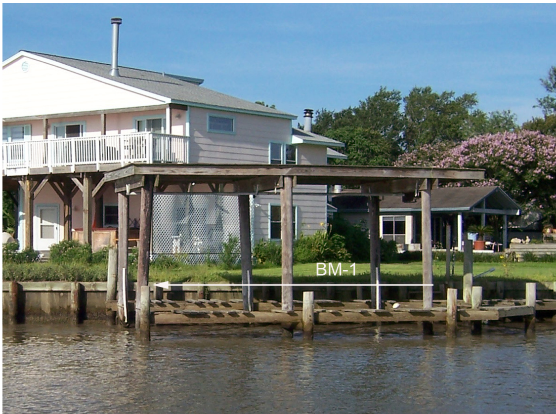
Figure 19. Picture of the boat dock used as the benchmark for the survey. Arrow labeled BM-1 shows the top of the pile used for the benchmark in this survey. Photo taken August 2006.
