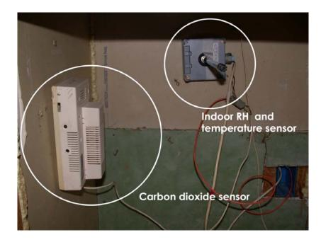
Figure 4.9 Indoor temperature / relative humidity sensor and carbon dioxide sensor
