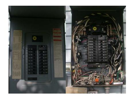
Figure 4.17 Electrical panel with the current transducers, face on (left) and face off (right)
