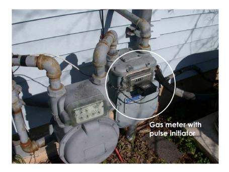
Figure 4.14 Gas meter with pulse initiator
