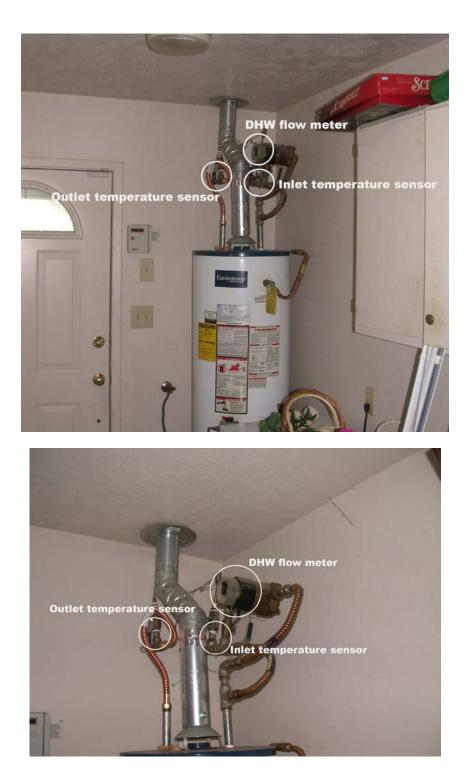
Figure 4.15 Flow meter attached to the domestic hot water heater
