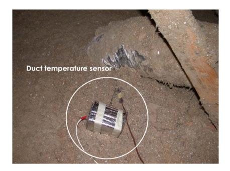
Figure 4.12 Duct temperature sensor with insulation
