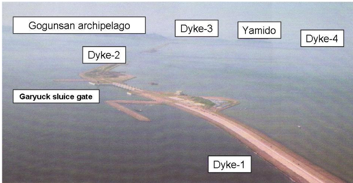
Figure 27 An aerial photo of the all construction works in the Saemangeum Project [from KARICO (2005).]
