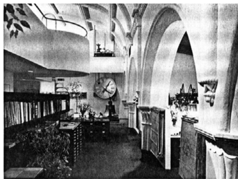
FIGURE 31. The Charles Street Meeting House (Interior view of office lobby) 68
