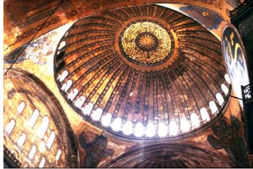
FIGURE 9. Hagia Sophia (Dome and openings) 40
