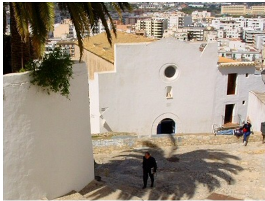
FIGURE 22. The Hospitalet Church (Exterior view) 59
