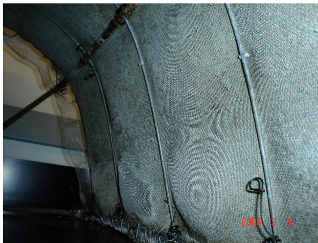
Fig. 37. Window screen sag
