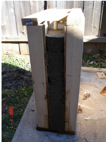
Fig. 30. Papercrete in wall panel form
