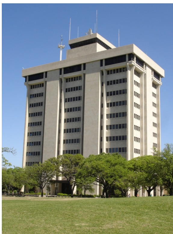
Figure 43. Eller O&M Building
