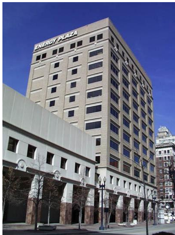
Figure 35. OPPD Energy Plaza East Building
