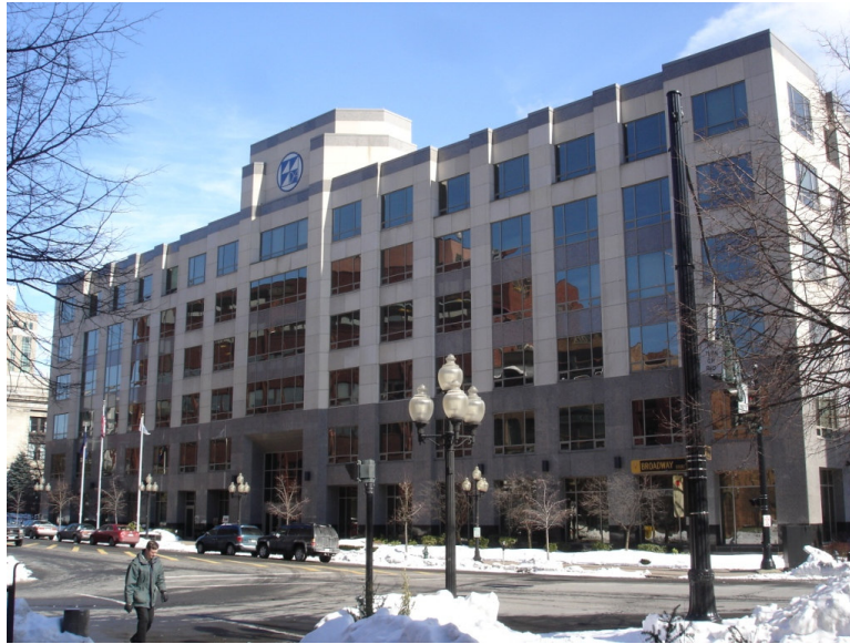
Figure 32. DASNY Corporate Headquarters Building
