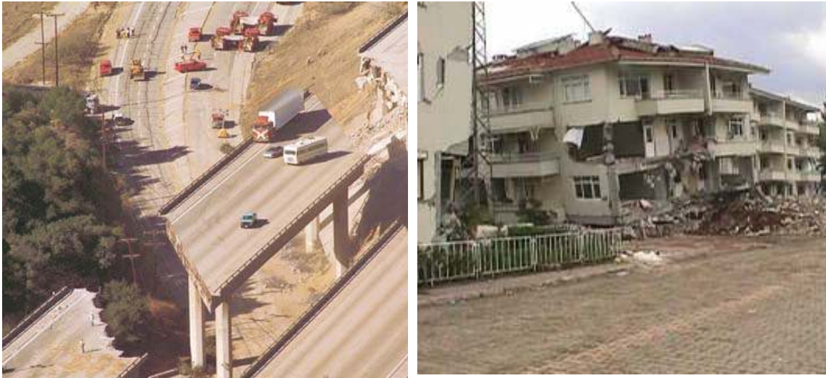
Fig. 1. Damage to a bridge and residential housing after (a) Northridge (1994) and (b) Izmit (1999) earthquakes
