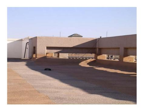
Fig. 12. Shadow: Bumpy. The curved edge of the shadow indicates bubbles in the roof sheathing. (Digital photograph © Jill Mulholland 2006).
