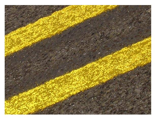
Fig. 45. Glow: Enlarging. The tiny glass spheres reflect and magnify light back. (Digital photograph © Jill Mulholland 2006).
