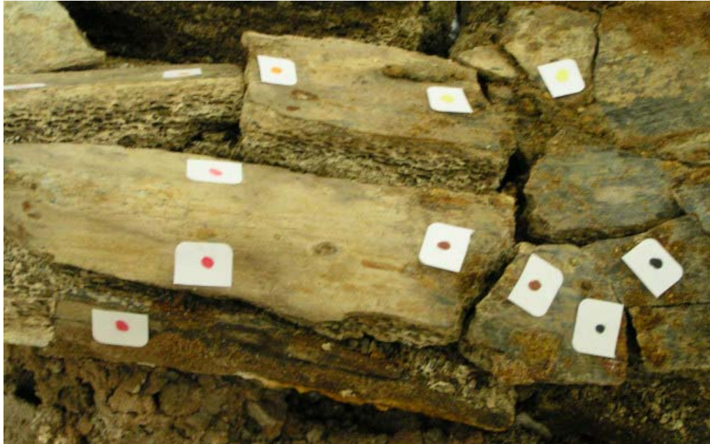
Figure 4.3. Marking the radius before taking it apart piece by piece.
