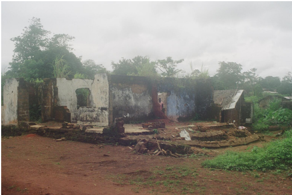
Figure 53: Remains of a Destroyed House in Koindu
