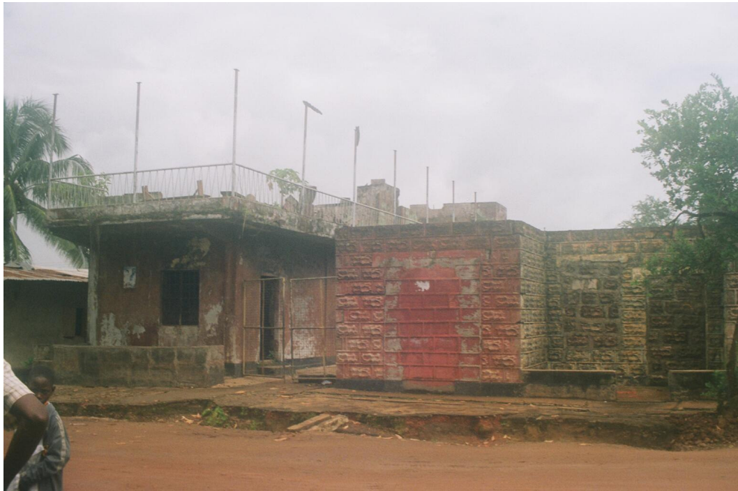
Figure 33: Remains of a Destroyed House in Kenema
