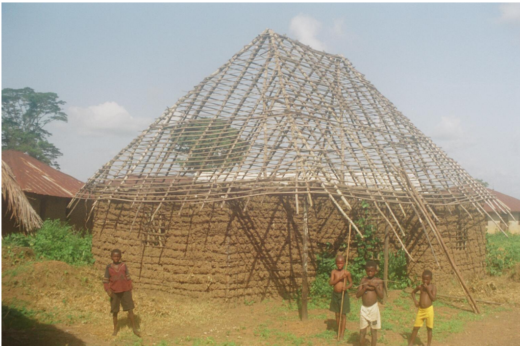
Figure 47: A House Under Construction in Yendema (Njaluahun Chiefdom)
