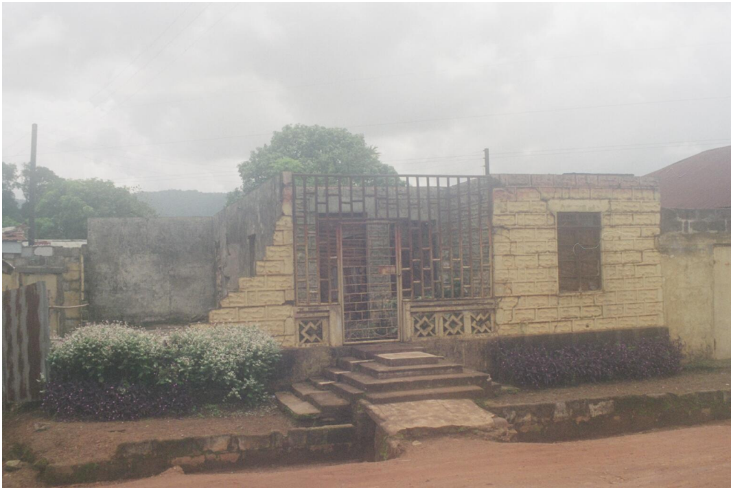
Figure 21: The Remains of an Important House in Kenema
