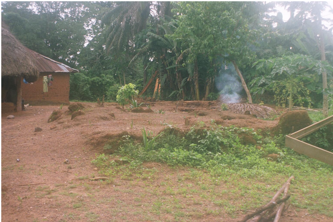
Figure 11: Remains of a House Foundation (Baiama II, Small Bo Chiefdom)
