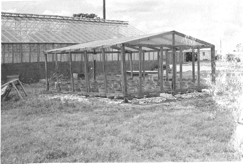
Figure 4. Shed shown with wall panels removed.
