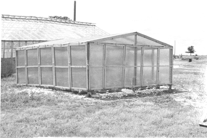
Figure 5. Shed shown with wall panels in place.
