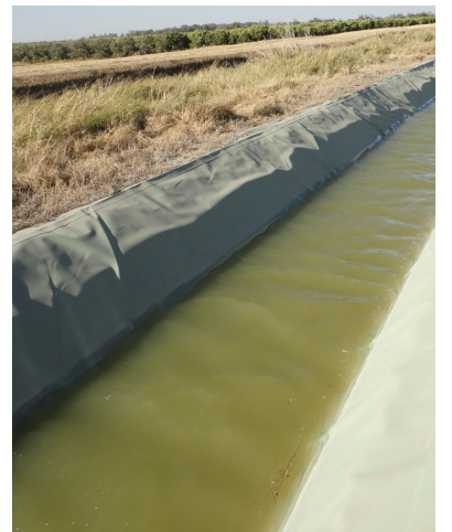
(TOP) Canal gate (BOTTOM) Canal-lining evaluation
