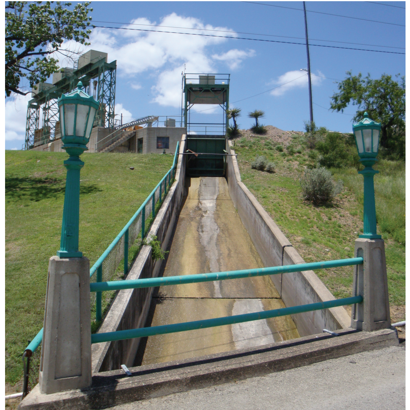
Spillway from the Maverick County Irrigation District main canal
