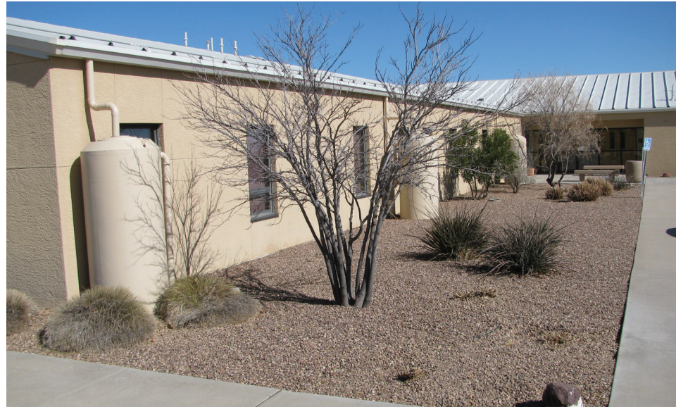
Rainwater harvesting tank demonstration
