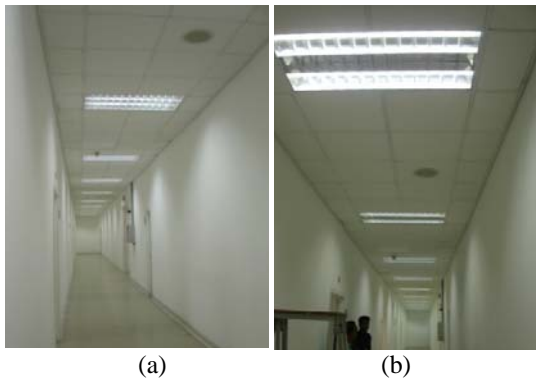
Figure 1. A corridor at LTC building (a) before (b) after delamping.
