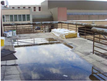
Fig. 2 – Site location of plots. The green roof boxes are located on a one-story patio with its own drainage problem.
