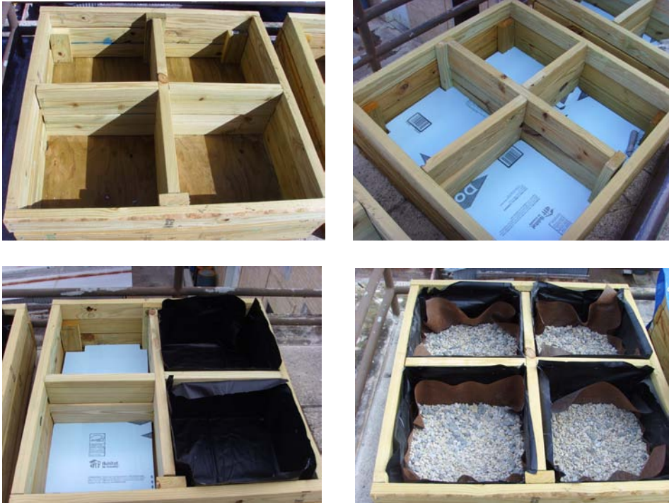
Fig. 3 – Construction of green roof plots. Clockwise from top left: frame, insulation layers, insolation and waterproofing and drainage layer.
